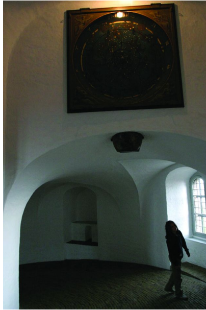
Figure 7. Accessing the tower via the ramp. Along the outer wall, the ramp has a length of 257.5 meters and a grade of 10%; long the inside wall the ramp is only 85.5 meters long, but with a grade of 33%. Both photographs by David A. Katz.
