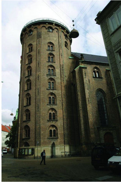
Figure 6. The Rundetårn illustrating its attachment to the adjacent building.
